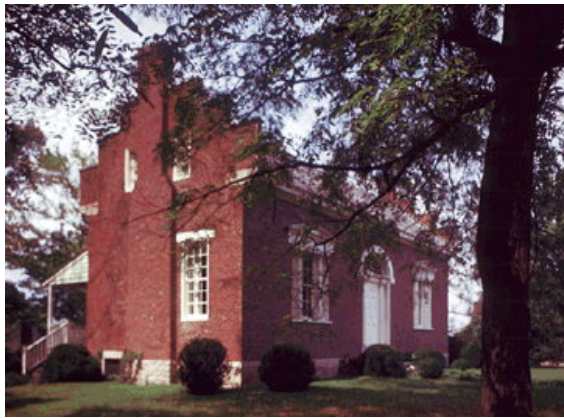
Carter House, Franklin, TN— National Historic Landmark
